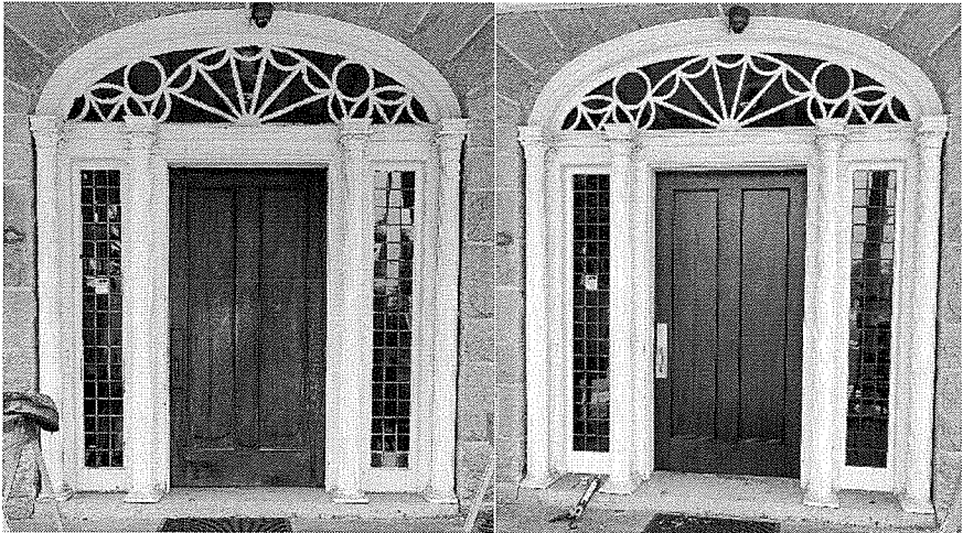
The original worn front door and windows.
